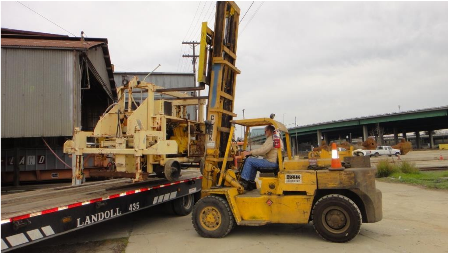
Meanwhile, back at the Shops, Alan operates the big yellow forklift to unload the tie-exchanger.
