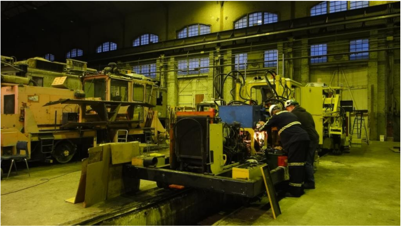
Scott and Frank troubleshooting issues with the Tie Shear
