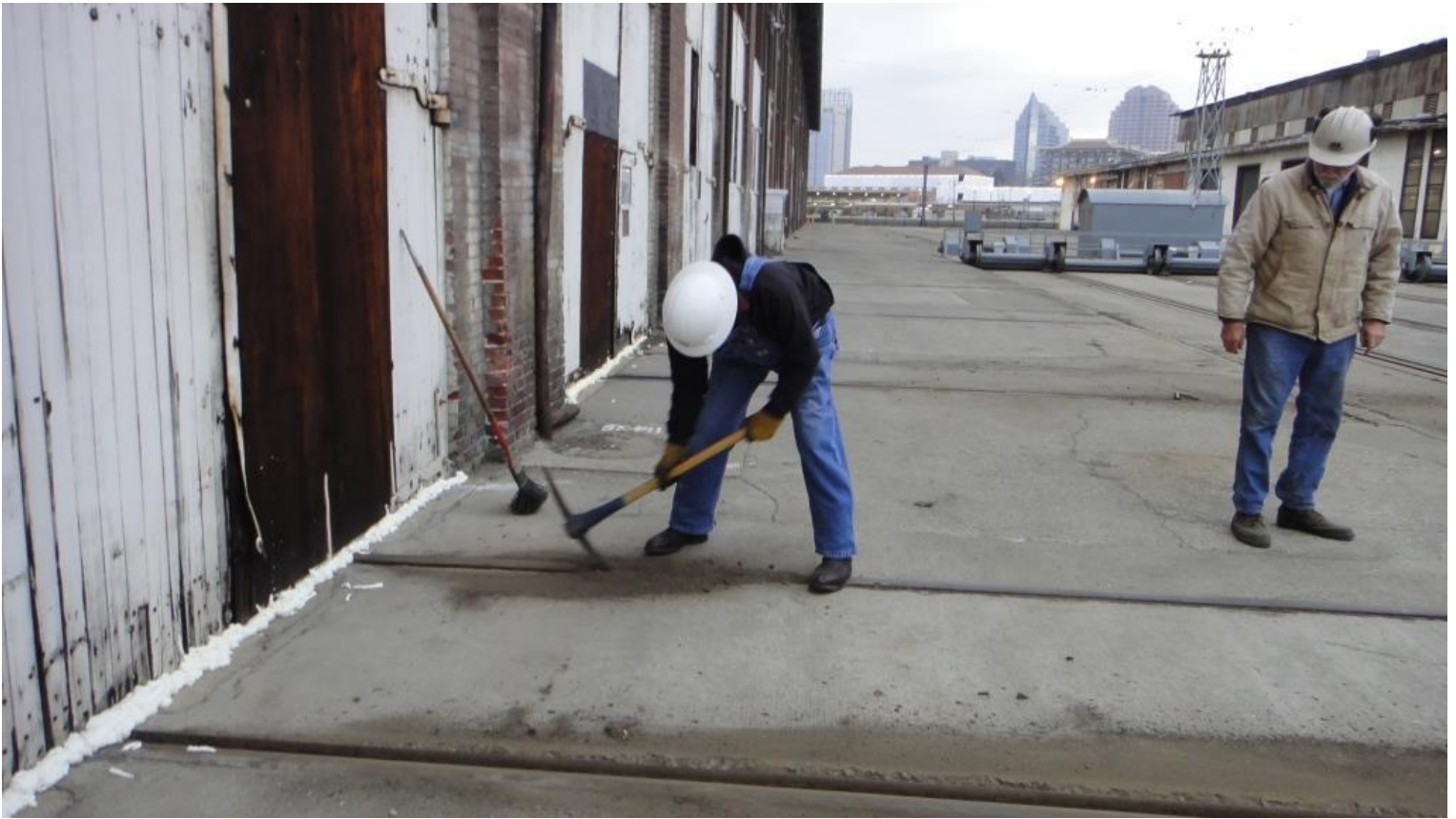
Cliff and Alan dig out the flange-ways along the apron of the Erecting Shop in preparation for Storm-a-saurus
