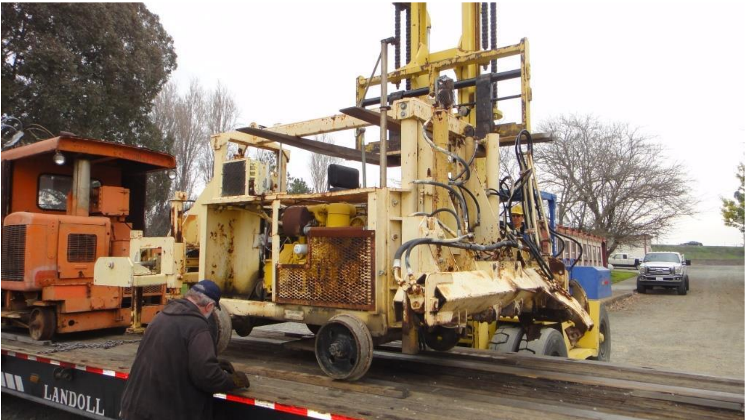
Frank guides the Jackson 125 tie-exchanger onto the flatbed truck.
